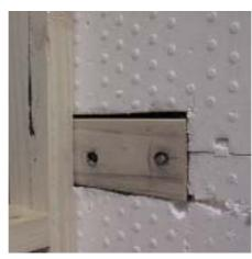
the concrete infill via cast in M12 bolts. (see Technical Manual page 78). Internal Superform BIG Block walls joining exterior Superform BIG Block walls are connected by forming a continuous concrete infill joint and providing L shaped reinforcing bars with adequate returns. A vertical reinforcing bar must be placed at the inside bend of the L bars (see Technical Manual page 77).
